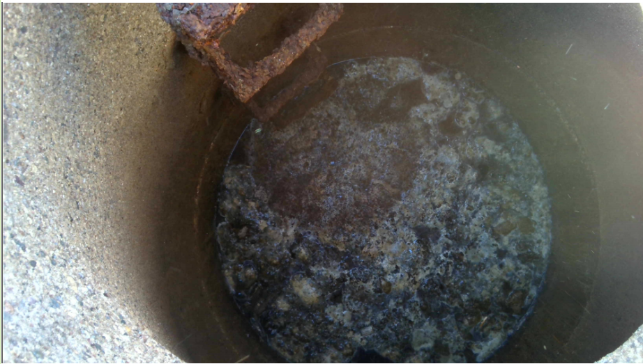
Wastewater Back-up in Manhole
