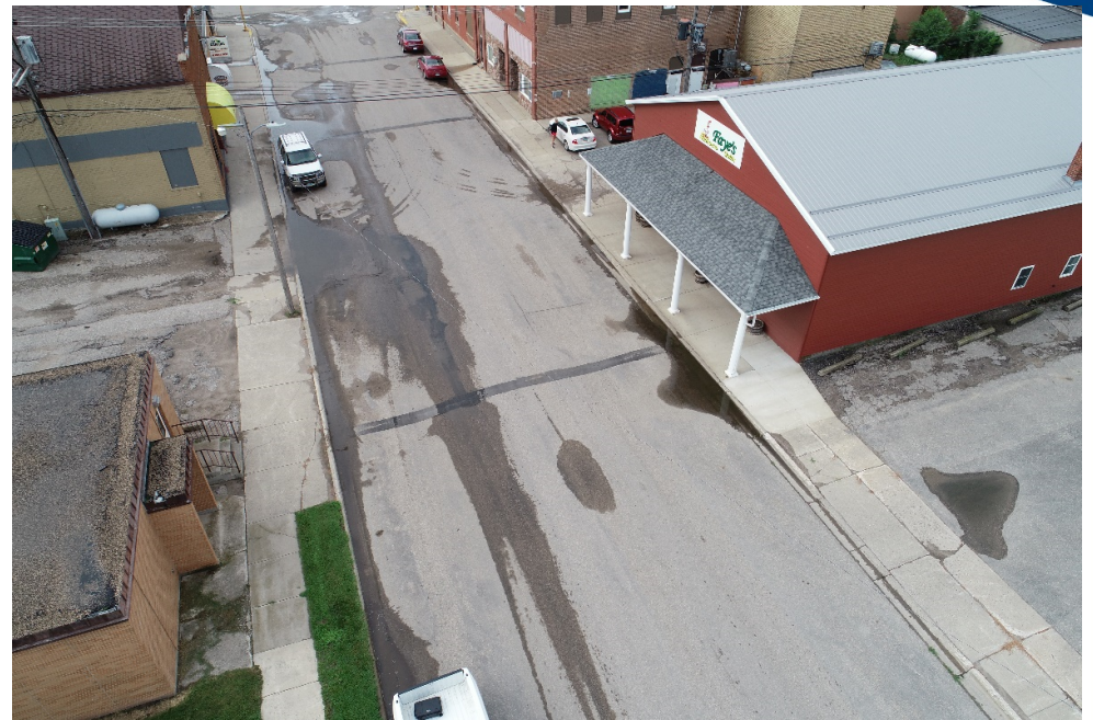
Water Ponding in Streets
